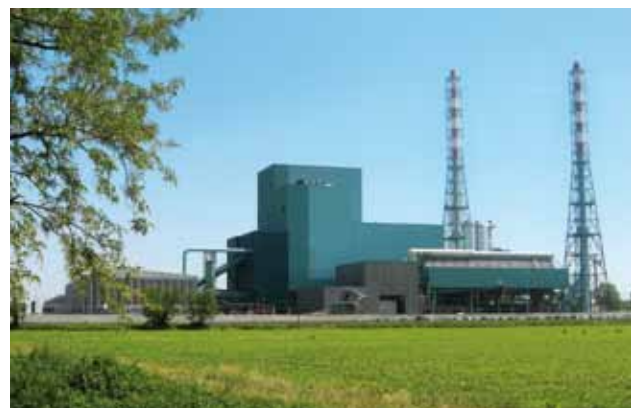
Incinerator - Courtesy of Lomellina Energia
