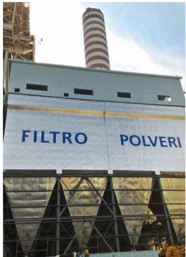
Power Plant Torrevaldaliga Nord ENEL - Courtesy of Termokimik
